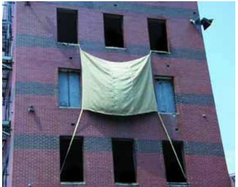
HOT•STOP 1500 HIGH RISE FIRE CURTAIN BEING DEPLOYED AT THE FDNY'S RANDALLS ISLAND TRAINING FACILITY.
